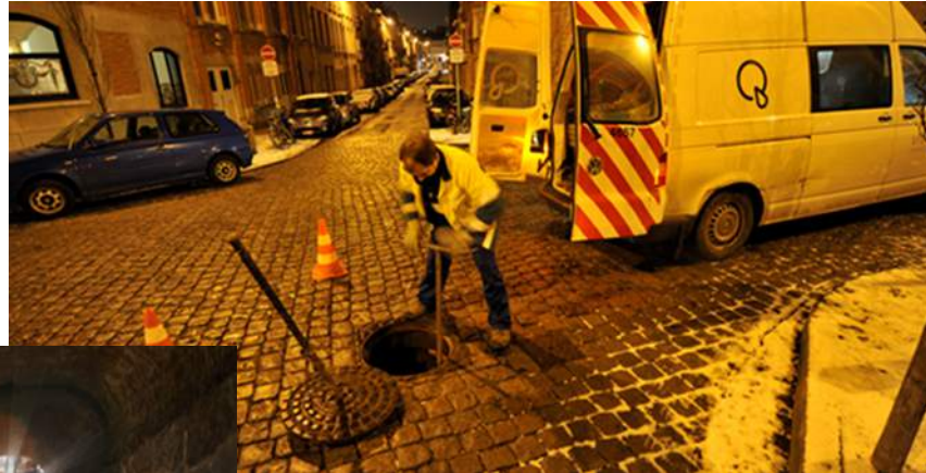
Distribution eau potable
